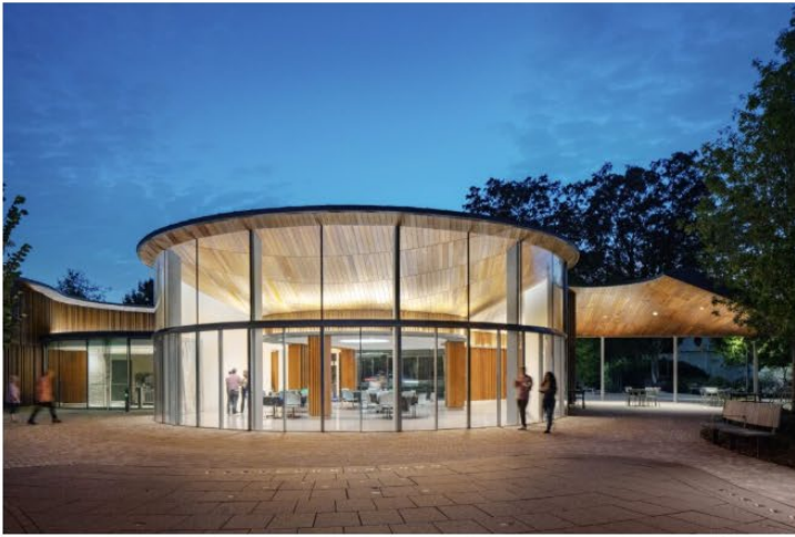
Despite the complex roof forms, the pavilions use standard building materials and dimensional lumber for the ceilings and exterior cladding.
